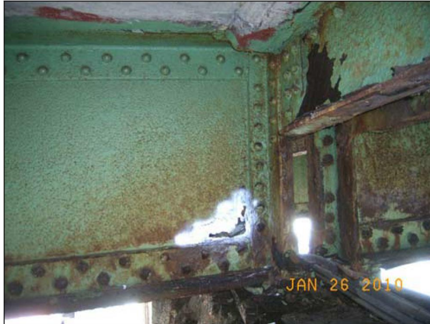
Main Bridge Photo 60 <09988a>: Span 1 Girder G4, Right side, at Pier 1. Large hole in web plate.
