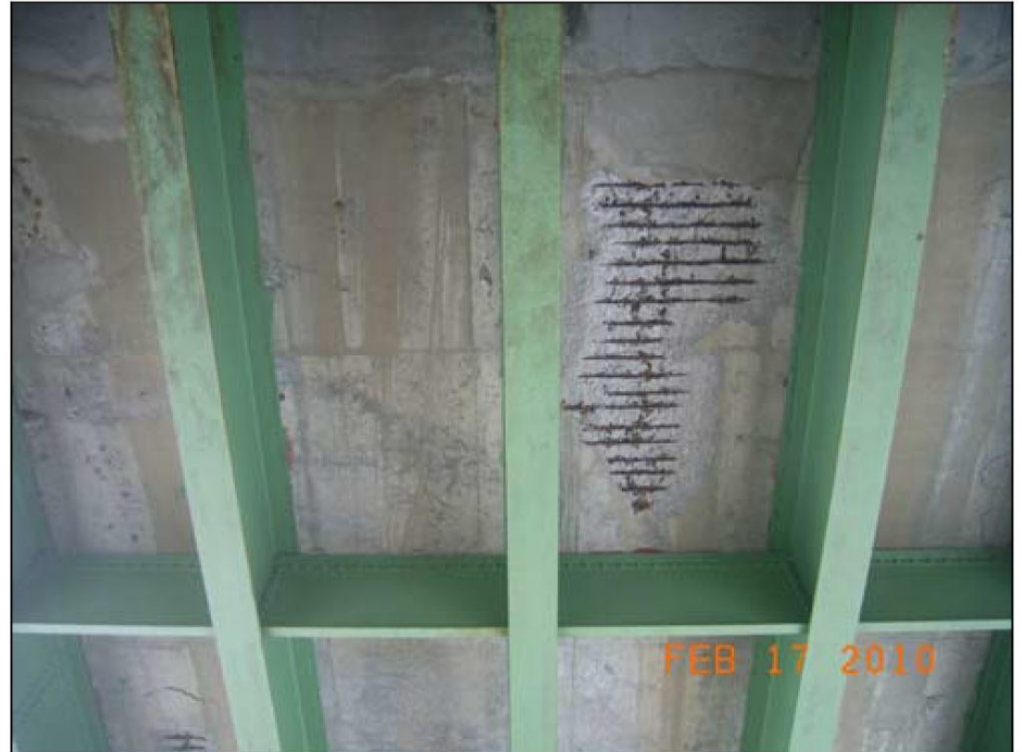
Ramp Bridge Photo 21 <Span 2 at Begin. Locally serious deck deterioration.
