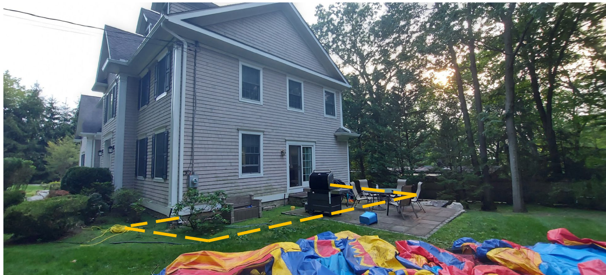
Side Yard: Dashed lines indicate extents of proposed wood deck at door sill level
