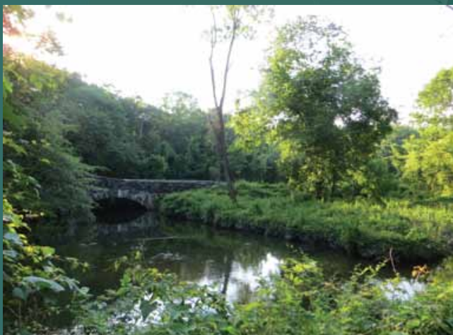
View west from Trailway bridge
