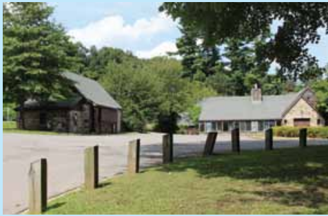
Existing driveway and unused buildings
