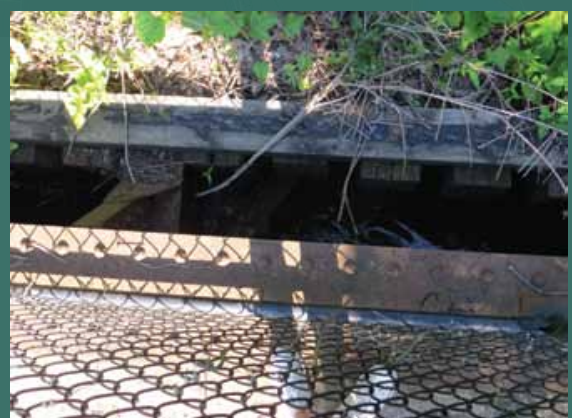
Railroad ties on Trailway bridge
