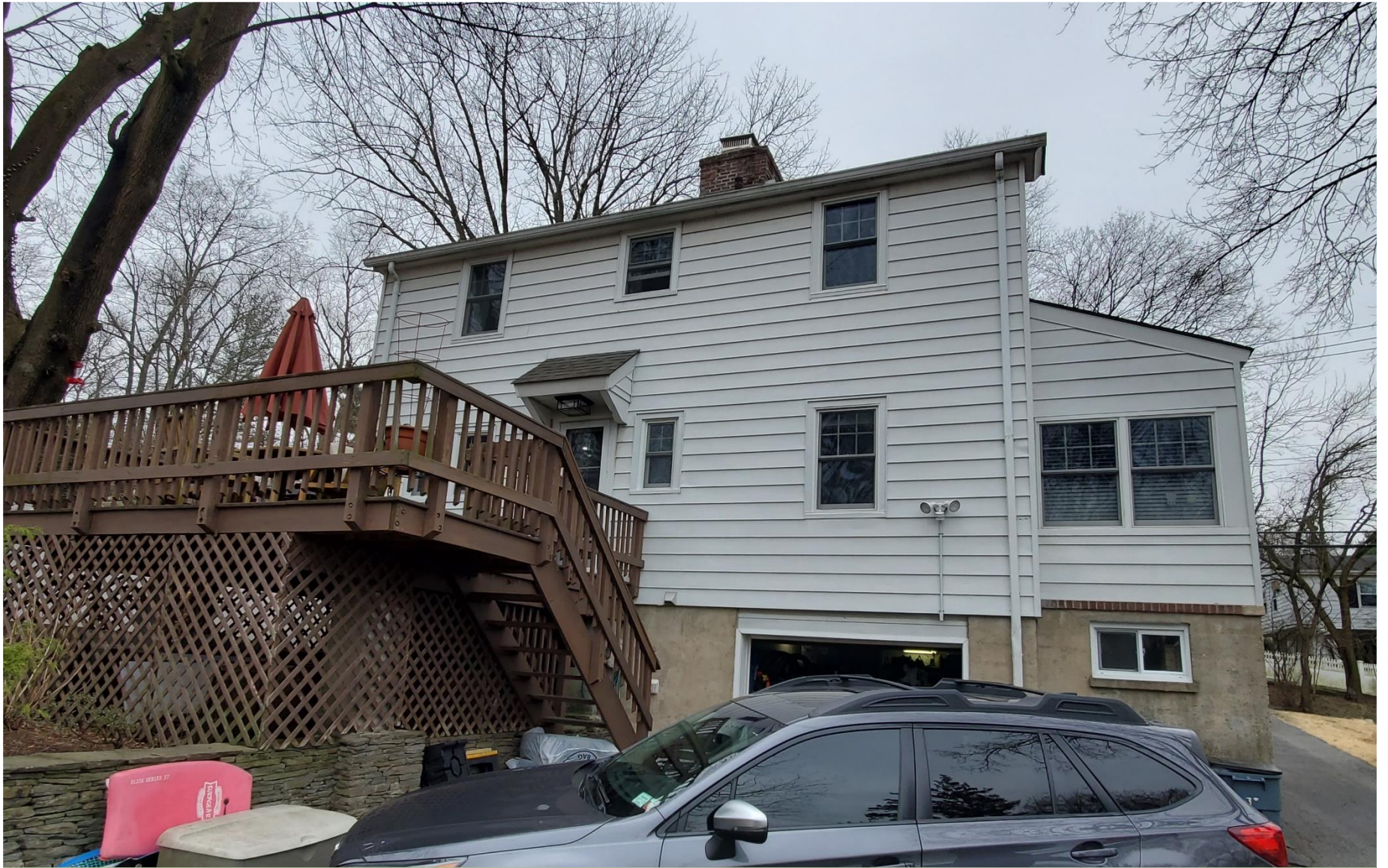
38 Heatherdell Road – Area of Proposed Construction
