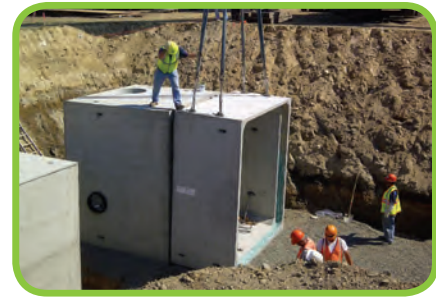
Modular Vault Assembly
