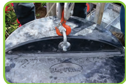
Cartridge Hoist Point
