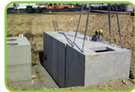
Vault End Section
