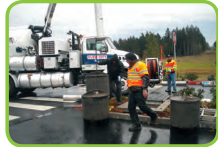
BayFilter System Cleanout
