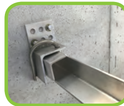
Hold Down Bar and Bracket
