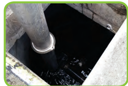
Jet Vactoring Through Access Hatch
