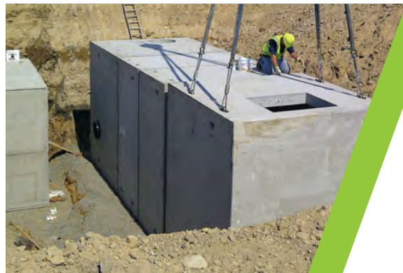
Vault End Section
