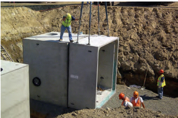
Modular Vault Assembly
