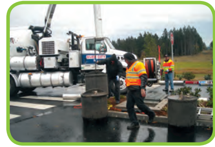
BayFilter System Cleanout
