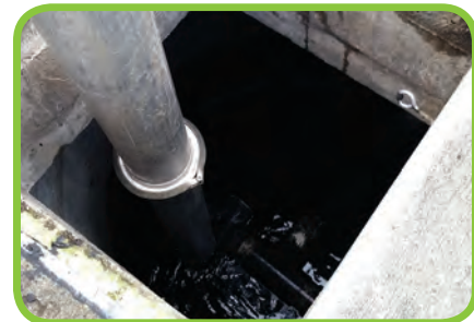
Jet Vactoring Through Access Hatch
