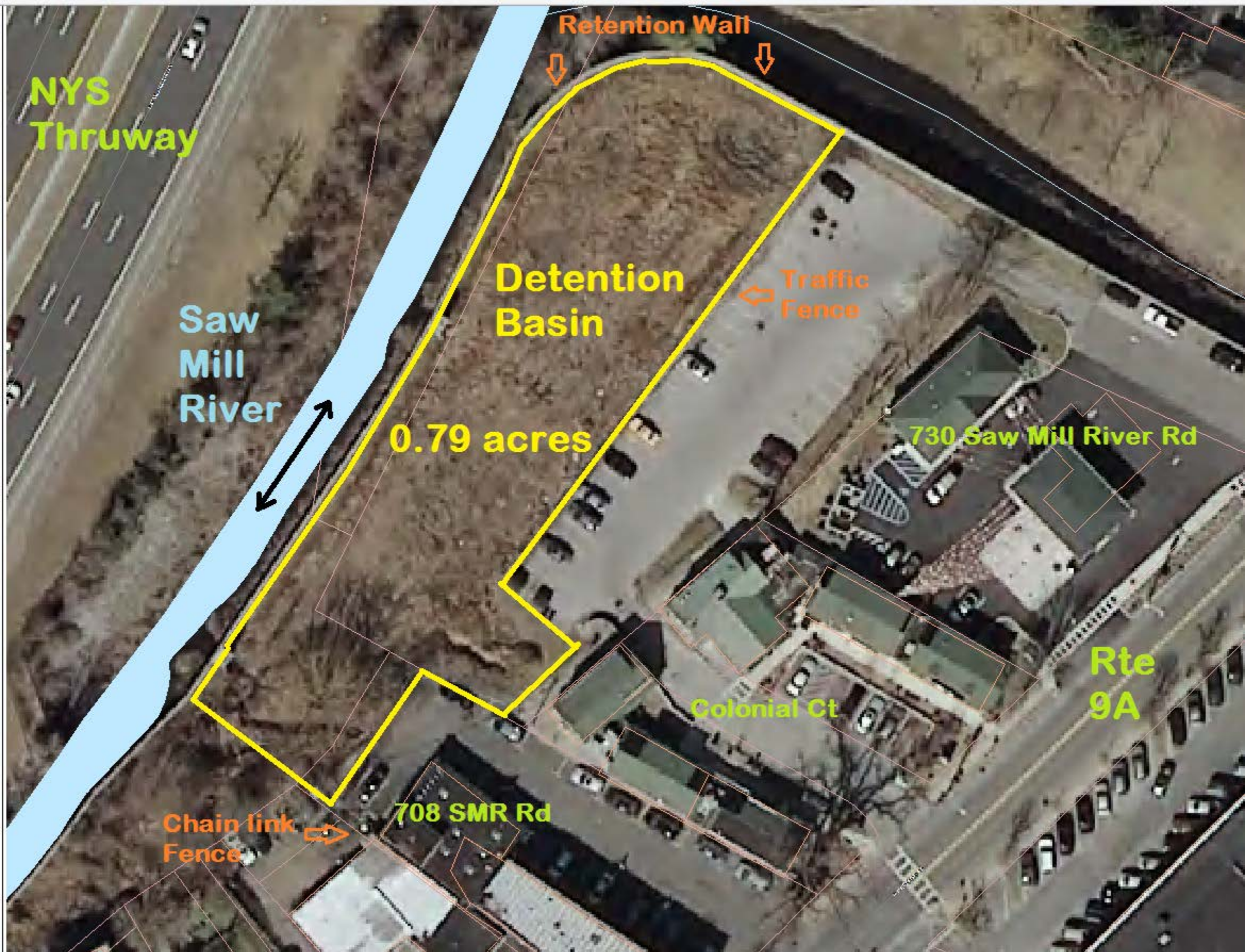
Figure A: Ardsley Detention Basin
