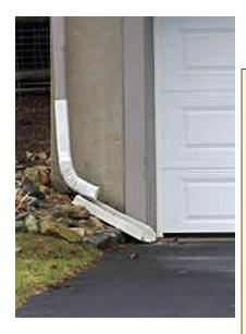
Some drain pipes run across your property right to edge, and discharge runoff directly into the street or onto the driveway. Not only does the flow pick up pollutants which go right to the storm drain, but a serious icing hazard is created in the winter. Village of Ardsley has an ordinance which prohibits this discharge due to the hazard it creates (see 156-2 below).
