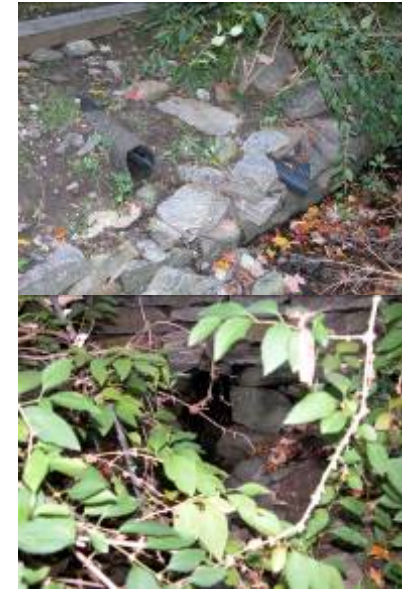
OF37: N 41 00 0.335 W 73 50 0.836 18" d rusted steel, bottom missing, 3' to top, obscured by veg., swift, no smell 2 X 4" d black corr at surface, dry 6" d asbestos at surface, dry
