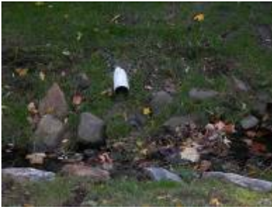
OF33: N 41 00 0.360 W 73 50 0.842 4" d white PVC at surface, dry
