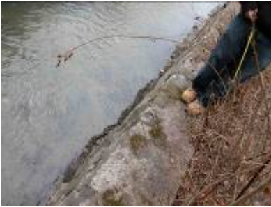
OF72: N 41 00 0.371 W 73 50 0.103 4"d black metal, 5" to top dry, in stone wall
