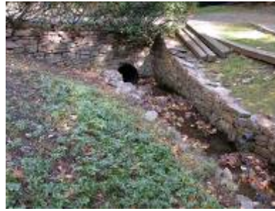
OF35: N 41 00 0.348 W 73 50 0.838 2' d black corr, 3' to top, moderate flow, collapsed stone wall obstruction 4" d black PVC, 1' to top, dry
