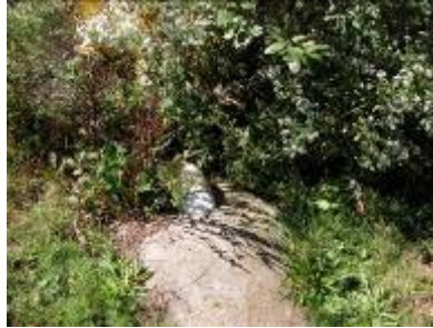
OF5: N 41 01 0.119 W 73 49 0.964 7''d white PVC elbow at surface, anchored in cement, dry, tall veg. covering
