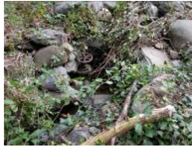
OF14: N 41 01 0.081 W 73 49 0.927 4"d iron pipe and valve 3' to top, very rusty, steady flow of stream, clear & clean
