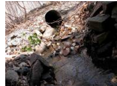
OF112: N 41 00 0.742 W 73 50 0.446 1'd metal corr, at surface 6" deep, swift, clean & clear
