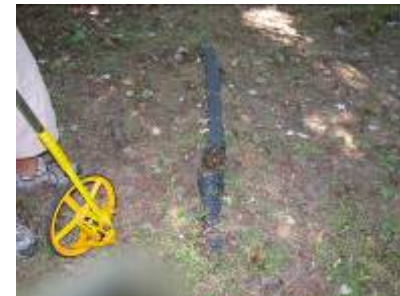
OF8: N 41 01 0.113 W 73 49 0.987 4''d white PVC, 4''d black corr plastic at surface, dry black pipe broken at 25' northwest (N 0.127 W 0.996)
