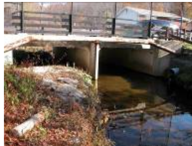
OF49: N 41 00 0.255 W 73 50 0.145 24' wide bridge, west silt, east clear 1' deep
