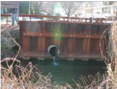
OF47: N 41 00 0.255 W 73 50 0.133 3'd corr steel, slight rust, 5' to top, clear & clean
