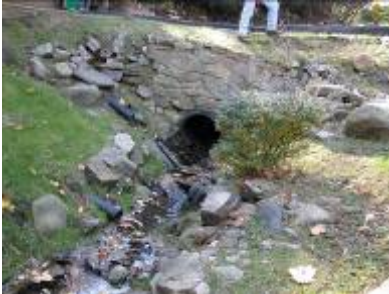
OF34: N 41 00 0.355 W 73 50 0.843 2' d black corr, 3' to top, swift 3 X 4" d white PVC at surface, dry some leaves
