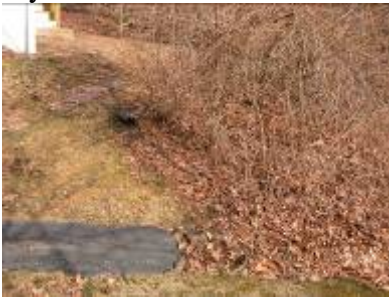
OF98: N 41 00 0.530 W 73 50 0.110 4" black corr, at surface leads to swale which leads to stream, dry
