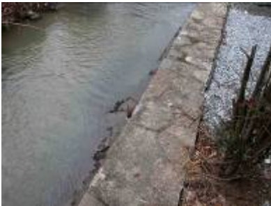
OF71: N 41 00 0.371 W 73 50 0.103 4"d rusted steel, 5" to top dry, in stone wall
