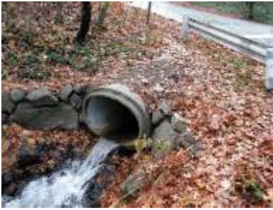
OF58: N 41 00 0.614 W 73 50 0.818 30" X 40" cement ellipse at surface, very swift, clean & clear
