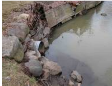
OF70: N 41 00 0.352 W 73 50 0.131 3'd steel corr, 3' to top 5" deep, flowing east to stream 4"d white PVC, 3' to top dry, on north side
