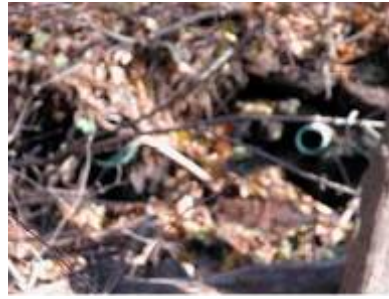
OF60: N 41 00 0.639 W 73 50 0.813 6'd white PVC, 5' to top dry 1'd green plastic, 5' to top dry
