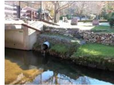
OF50: N 41 00 0.255 W 73 50 0.145 3'd steel pipe, 3' to top, steady flow
