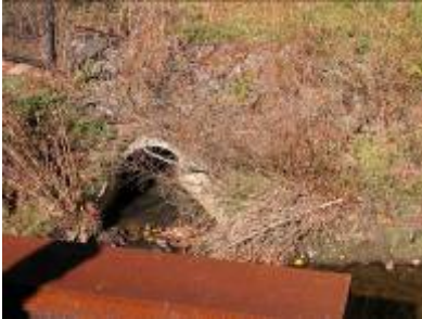
OF46: N 41 00 0.255 W 73 50 0.133 3'd cement, at surface, 1' deep, some muck
