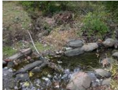
OF15: N 41 01 0.076 W 73 49 0.915 1/2" PVC (UL listed) at surface, no outlet, stream is clean & clear, water depth 8"
