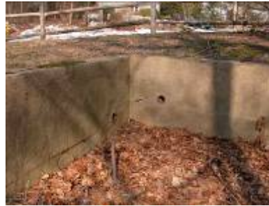
OF100: N 41 00 0.550 W 73 50 0.119 4" d clay, 2' to top in cement wall, dry part of old drain system
