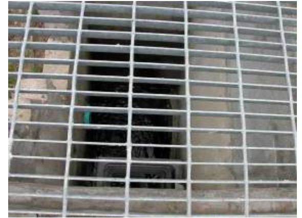
OF181 N 41 01 0.303 W 73 50 0.636 East side: 1'd green PVC, 4' to top, steady flow to west, no smell West side: 3'd black corr PVC, 10' to top, receiving flow Catch basin beneath
