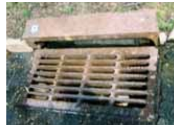
SD74: N41°00.376'W73°51.042' Standing water, slight debris, sewage odor
