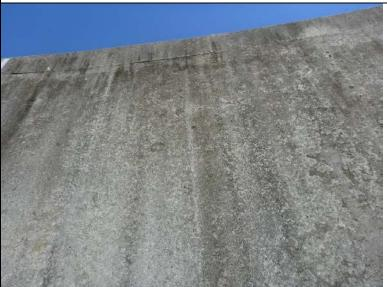
**Inspect ID:** NAR1\_2019\_a\_0032 **Title:** USACE\_CENAN\_NAR1\_2019\_a\_0032\_2.jpg **Rated Item:** 4. Concrete Surfaces **Caption:** Rating: Minimally Acceptable; Remarks: Apparent construction joint has opened along the top of the protected side of monoliths 39 and 40.; Action: Fill the crack and repair concrete surface in accordance with USACE guidelines.; Station\_1: 7+80U
