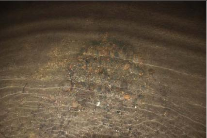
Inspect ID: NAR1\_2019\_a\_0061 Title: USACE\_CENAN\_NAR1\_2019\_a\_0061\_1.jpg Rated Item: 5. Concrete Surfaces Caption: Rating: Minimally Acceptable; Remarks: Scour hole at bottom of concrete channel. Could not access in 2019.; Action: Repair concrete surfaces in accordance with USACE guidelines.; Station\_1: 1+45U; Photo taken prior to the 2019 inspection.
