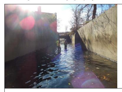
Inspect ID: NAR1\_2019\_a\_0076 Title: USACE\_CENAN\_NAR1\_2019\_a\_0076\_1.jpg Rated Item: 2. Shoaling (sediment deposition) Caption: Rating: Minimally Acceptable; Remarks: Shoaling in channel between monoliths 13 and 14. Could not access in 2019.; Action: Remove sediment in accordance with USACE guidelines.; Station\_1: 3+15U; Photo taken prior to the 2019 inspection.
