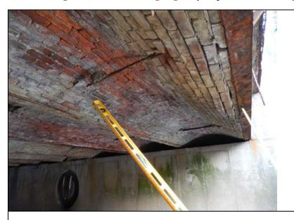
Inspect ID: NAR1\_2019\_a\_0062 Title: USACE\_CENAN\_NAR1\_2019\_a\_0062\_2.jpg Rated Item: 3. Encroachments Caption: Rating: Minimally Acceptable; Remarks: Bricks of the vaulted ceiling, beneath the old bridge, are about to fall due to corroded and broken tie rods. Falling debris could obstruct the channel. Could not observe in 2019.; Action: Shoring is needed to prevent failure of the vaulted ceiling and original bridge structure.; Station\_1: 1+35U; Photo taken prior to the 2019 inspection.
