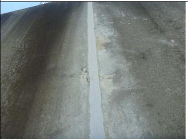
Inspect ID: NAR1\_2019\_a\_0026 Title: USACE\_CENAN\_NAR1\_2019\_a\_0026\_1.jpg Rated Item: 4. Concrete Surfaces Caption: Rating: Minimally Acceptable; Remarks: Minor spalling on the protected side of monolith 47 near joint.; Action: Repair concrete surface in accordance with USACE Guidelines.; Station\_1: 2+20B
