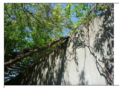
Inspect ID: NAR1\_2019\_a\_0054 Title: USACE\_CENAN\_NAR1\_2019\_a\_0054\_1.jpg Rated Item: 1. Unwanted Vegetation Growth Caption: Rating: Minimally Acceptable; Remarks: Vegetation on top of floodwall at monolith 12.; Action: Remove vegetation in accordance with USACE guidelines.; Station\_1: 2+50U
