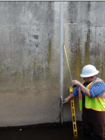
Inspect ID: NAR1\_2019\_a\_0066 Title: USACE\_CENAN\_NAR1\_2019\_a\_0066\_1.jpg Rated Item: 4. Concrete Surfaces Caption: Rating: Minimally Acceptable; Remarks: Spalling at joint between monoliths 5 and 4. Could not access in 2019.; Action: Repair concrete surface in accordance with USACE Guidelines.; Station\_1: 0+85U; Photo taken prior to the 2019 inspection.
