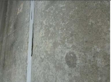
Inspect ID: NAR1\_2019\_a\_0037 Title: USACE\_CENAN\_NAR1\_2019\_a\_0037\_1.jpg Rated Item: 4. Concrete Surfaces Caption: Rating: Minimally Acceptable; Remarks: Small spall on protected side of monolith 30 at joint with monolith 29.; Action: Repair concrete surface in accordance with USACE Guidelines.; Station\_1: 5+90U
