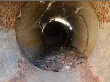
**Inspect ID:** NAR1\_2019\_a\_0052 **Title:** USACE\_CENAN\_NAR1\_2019\_a\_0052\_2.jpg **Rated Item:** 2. Encroachments **Caption:** Rating: Minimally Acceptable; Remarks: Unauthorized flap gate in monolith 18 is connected to 8" IDP noted in observation #50. Flap gate found in open position in 2016.; Action: Maintian flap gate. Investigate easement agreement and dispose of encroachment accordingly.; Station\_1: 3+75U; Photo taken prior to the 2019 inspection.
