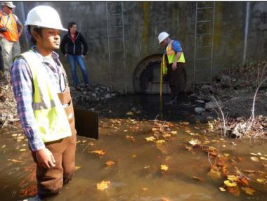
Inspect ID: NAR1\_2019\_a\_0041 Title: USACE\_CENAN\_NAR1\_2019\_a\_0041\_1.jpg Rated Item: 11. Flap Gates/ Flap Valves/ Pinch Valves Caption: Rating: Minimally Acceptable; Remarks: Flap gate of DS#3 is blocked by sediment deposition. Could not access in 2019.; Action: Remove sediment in accordance with USACE guidelines.; Station\_1: 5+15U; Photo taken prior to the 2019 inspection.
