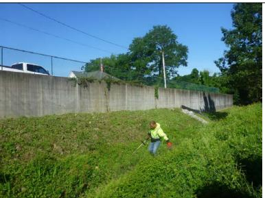
Inspect ID: NAR1\_2019\_a\_0004 Title: USACE\_CENAN\_NAR1\_2019\_a\_0004\_1.jpg Rated Item: 2. Encroachments Caption: Rating: Minimally Acceptable; Remarks: Fence on top of floodwall running from monolith 47-60 not in the original plans.; Action: Seek authorization from USACE for the encroachment to remain.; Station\_1: 2+20B; Station\_2: 4+45B
