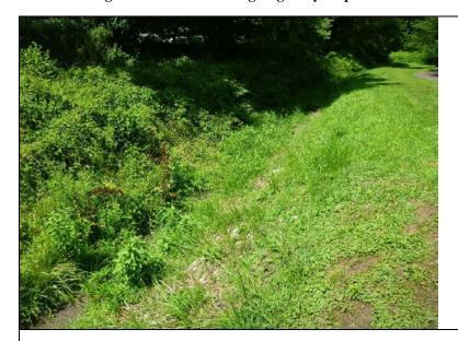
Inspect ID: NAR1\_2019\_a\_0086 Title: USACE\_CENAN\_NAR1\_2019\_a\_0086\_1.jpg Rated Item: 1. Vegetation and Obstructions Caption: Rating: Minimally Acceptable; Remarks: Sediment and vegetation obstructing flow in Interceptor Ditch #1.; Action: Remove sediment and vegetation in accordance with USACE guidelines.; Station\_1: 0+00A; Station\_2: 5+00A
