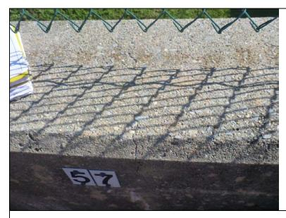
Inspect ID: NAR1\_2019\_a\_0015 Title: USACE\_CENAN\_NAR1\_2019\_a\_0015\_1.jpg Rated Item: 4. Concrete Surfaces Caption: Rating: Minimally Acceptable; Remarks: Minor cracking and efflorescence at the top of monolith 57.; Action: Monitor cracking and efflorescence to ensure they do not worsen. Repair concrete in accordance with USACE guidelines as necessary.; Station\_1: 4+05B
