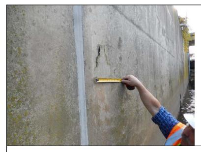
Inspect ID: NAR1\_2019\_a\_0071 Title: USACE\_CENAN\_NAR1\_2019\_a\_0071\_1.jpg Rated Item: 4. Concrete Surfaces Caption: Rating: Minimally Acceptable; Remarks: Spalling at monolith 5 near joint of monolith 6. Could not access in 2019.; Action: Repair concrete surface in accordance with USACE Guidelines.; Station\_1: 1+05U; Photo taken prior to the 2019 inspection.
