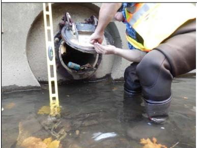
Inspect ID: NAR1\_2019\_a\_0069 Title: USACE\_CENAN\_NAR1\_2019\_a\_0069\_2.jpg Rated Item: 11. Flap Gates/ Flap Valves/ Pinch Valves Caption: Rating: Minimally Acceptable; Remarks: DS#1. Flap gate operated in 2016, but stiffly. Sediment in the way. Could not access in 2019.; Action: Clean DS#1 and lubricate flap gate.; Station\_1: 0+40U; Photo taken prior to 2019 inspection.
