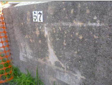
Inspect ID: NAR1\_2019\_a\_0015 Title: USACE\_CENAN\_NAR1\_2019\_a\_0015\_2.jpg Rated Item: 4. Concrete Surfaces Caption: Rating: Minimally Acceptable; Remarks: Minor cracking and efflorescence at the top of monolith 57.; Action: Monitor cracking and efflorescence to ensure they do not worsen. Repair concrete in accordance with USACE guidelines as necessary.; Station\_1: 4+05B
