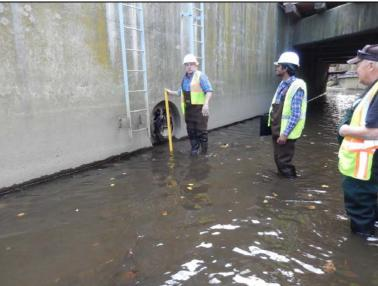
**Inspect ID:** NAR1\_2019\_a\_0067 **Title:** USACE\_CENAN\_NAR1\_2019\_a\_0067\_2.jpg **Rated Item:** 2. Shoaling (sediment deposition) **Caption:** Rating: Minimally Acceptable; Remarks: Shoaling at DS#1 in flood reduction channel.; Action: Remove sediment from channel to ensure maximum flow capacity.; Station\_1: 0+55U; ;; Photo taken prior to 2019 inspection.
