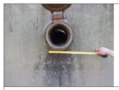
Inspect ID: NAR1\_2019\_a\_0052 Title: USACE\_CENAN\_NAR1\_2019\_a\_0052\_1.jpg Rated Item: 2. Encroachments Caption: Rating: Minimally Acceptable; Remarks: Unauthorized flap gate in monolith 18 is connected to 8" IDP noted in observation #50. Flap gate found in open position in 2016.; Action: Maintian flap gate. Investigate easement agreement and dispose of encroachment accordingly.; Station\_1: 3+75U; Photo taken prior to the 2019 inspection.
