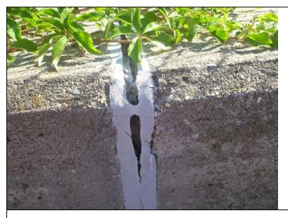
Inspect ID: NAR1\_2019\_a\_0016 Title: USACE\_CENAN\_NAR1\_2019\_a\_0016\_4.jpg Rated Item: 7. Monolith Joints Caption: Rating: Minimally Acceptable; Remarks: The gap sealant has cracked and separated in numerous joints along the entire length of the floodwall.; Action: Explore alternative joint stop material that can withstand the area's unique conditions. Clean joint and apply fresh sealant.; Station\_1: 0+00U; Station\_2: 4+45B
