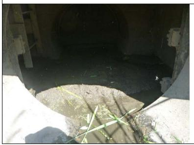
**Inspect ID:** NAR1\_2019\_a\_0034 **Title:** USACE\_CENAN\_NAR1\_2019\_a\_0034\_1.jpg **Rated Item:** 10. Sluice/ Slide Gates **Caption:** Rating: Minimally Acceptable; Remarks: DS # 4 sluice gate operated during 2016 inspection. Cannot fully close due to sediment at bottom of structure. NYSDEC plans to replace the crank with an electric motor.; Action: Remove sediment and debris.; Station\_1: 6+85U; ;;
