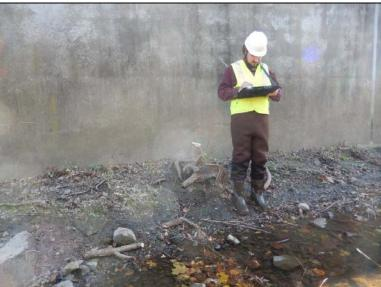
Inspect ID: NAR1\_2019\_a\_0036 Title: USACE\_CENAN\_NAR1\_2019\_a\_0036\_1.jpg Rated Item: 2. Encroachments Caption: Rating: Minimally Acceptable; Remarks: Stumps and tree limbs adjacent to exposed face of floodwall. Could not access in 2019.; Action: Remove debris and stumps.; Station\_1: 6+10U; Photo taken prior to the 2019 inspection.
