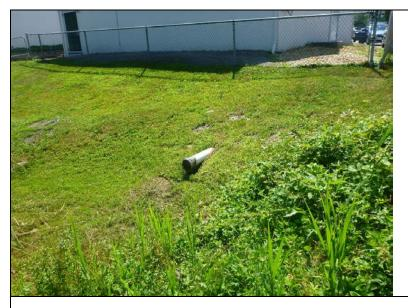
**Inspect ID:** NAR1\_2019\_a\_0046 **Title:** USACE\_CENAN\_NAR1\_2019\_a\_0046\_1.jpg **Rated Item:** 2. Encroachments **Caption:** Rating: Minimally Acceptable; Remarks: Two 8" PVC pipes that discharge in ponding area #2 are not shown on the project plans. Some erosion has occurred below the southernmost pipe; Action: Local sponsor should investigate and document the encroachments.; Station\_1: 5+15U;
