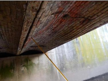
Inspect ID: NAR1\_2019\_a\_0062 Title: USACE\_CENAN\_NAR1\_2019\_a\_0062\_1.jpg Rated Item: 3. Encroachments Caption: Rating: Minimally Acceptable; Remarks: Bricks of the vaulted ceiling, beneath the old bridge, are about to fall due to corroded and broken tie rods. Falling debris could obstruct the channel. Could not observe in 2019.; Action: Shoring is needed to prevent failure of the vaulted ceiling and original bridge structure.; Station\_1: 1+35U; Photo taken prior to the 2019 inspection.
