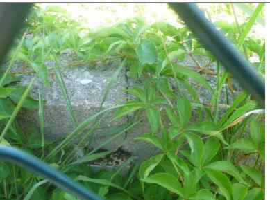
**Inspect ID:** NAR1\_2019\_a\_0006 **Title:** USACE\_CENAN\_NAR1\_2019\_a\_0006\_1.jpg **Rated Item:** 4. Concrete Surfaces **Caption:** Rating: Minimally Acceptable; Remarks: 1/4" crack across the top of monolith 59 associated with a piece of wood in the concrete.; Action: Remove wood blocking and patch concrete.; Station\_1: 4+45B
