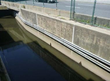
Inspect ID: NAR1\_2019\_a\_0072 Title: USACE\_CENAN\_NAR1\_2019\_a\_0072\_1.jpg Rated Item: 3. Encroachments Caption: Rating: Minimally Acceptable; Remarks: Metal conduits (pipes) on right wall of concrete channel.; Action: Investigate easement agreement and dispose of encroachment accordingly.; Station\_1: 0+90U
