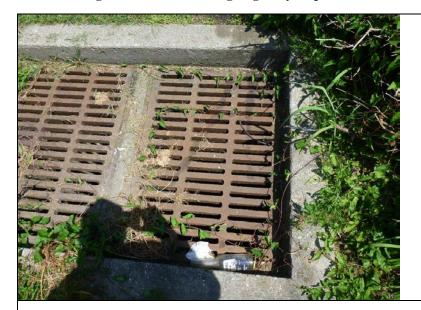
**Inspect ID:** NAR1\_2019\_a\_0081 **Title:** USACE\_CENAN\_NAR1\_2019\_a\_0081\_1.jpg **Rated Item:** 12. Trash Racks (non-mechanical) **Caption:** Rating: Acceptable; Remarks: Drop inlet #3 appears operable.; Action: Monitor conditions at the drop inlet.; Station\_1: 5+55A
