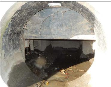
Inspect ID: NAR1\_2019\_a\_0034 Title: USACE\_CENAN\_NAR1\_2019\_a\_0034\_3.jpg Rated Item: 10. Sluice/ Slide Gates Caption: Rating: Minimally Acceptable; Remarks: DS # 4 sluice gate operated during 2016 inspection. Cannot fully close due to sediment at bottom of structure. NYSDEC plans to replace the crank with an electric motor.; Action: Remove sediment and debris.; Station\_1: 6+85U; ;; Photo taken prior to 2019 inspection.
