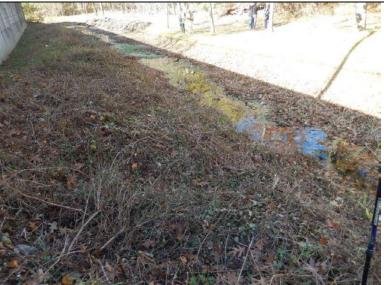
Inspect ID: NAR1\_2019\_a\_0020 Title: USACE\_CENAN\_NAR1\_2019\_a\_0020\_2.jpg Rated Item: 7. Foundation of Concrete Structures Caption: Rating: Minimally Acceptable; Remarks: Two large animal burrows on unprotected side of floodwall, 1-2 ft deep. Did not access in 2019.; Action: Eliminate burrowing animals; completely fill in burrows in accordance with USACE guidelines.; Station\_1: 3+30B; Photo taken prior to the 2019 inspection.
