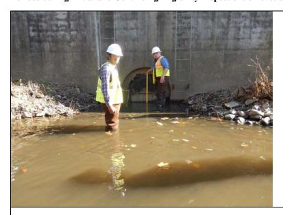
Inspect ID: NAR1\_2019\_a\_0035 Title: USACE\_CENAN\_NAR1\_2019\_a\_0035\_1.jpg Rated Item: 11. Flap Gates/ Flap Valves/ Pinch Valves Caption: Rating: Minimally Acceptable; Remarks: Flap gate of drainage structure #4 is partially blocked by sediment deposition. Could not access in 2019.; Action: Remove sediment in accordance with USACE guidelines.; Station\_1: 6+85U; Photo taken prior to the 2019 inspection.
