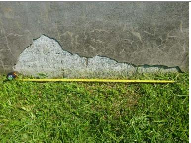
Inspect ID: NAR1\_2019\_a\_0029 Title: USACE\_CENAN\_NAR1\_2019\_a\_0029\_2.jpg Rated Item: 4. Concrete Surfaces Caption: Rating: Minimally Acceptable; Remarks: Concrete spalling on recently repaired areas on the protected side of the floodwall at the base of monoliths 39-42. Exposed rebar on 42. Heavy efflorescence on 41.; Action: Fill cracks and repair spalling in accordance with USACE guidelines.; Station\_1: 0+30B
