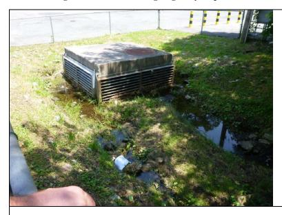
Inspect ID: NAR1\_2019\_a\_0080 Title: USACE\_CENAN\_NAR1\_2019\_a\_0080\_1.jpg Rated Item: 1. Vegetation and Obstructions Caption: Rating: Minimally Acceptable; Remarks: Sediment and vegetation partially blocking flow of the lower portion of interceptor ditch #2 at the blow-off tunnel connection. Sedimentation appeared improved over 2016 and the Village of Ardsley noted that they have cleaned it out before.; Action: Remove sediment in accordance with USACE guidelines.; Station\_1: 0+00C
