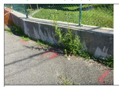
Inspect ID: NAR1\_2019\_a\_0012 Title: USACE\_CENAN\_NAR1\_2019\_a\_0012\_1.jpg Rated Item: 4. Concrete Surfaces Caption: Rating: Minimally Acceptable; Remarks: Gouging of the protected side of monoliths 57 and 58, may be the result of improper snow removal practices.; Action: The local sponsor should contact the property owner and advise them that the wall cannot be used as a push wall. Repair concrete surfaces in accordance with USACE guidelines.; Station\_1: 4+25B
