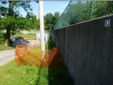
Inspect ID: NAR1\_2019\_a\_0018 Title: USACE\_CENAN\_NAR1\_2019\_a\_0018\_1.jpg Rated Item: 2. Encroachments Caption: Rating: Minimally Acceptable; Remarks: Utility pole and guy wire within 4 ft of floodwall on protected side. NYSDEC indicated that there are plans to move the pole and wire across the drive during a future upgrade.; Action: Proceed with the plan to move the pole during the next upgrade.; Station\_1: 3+30B
