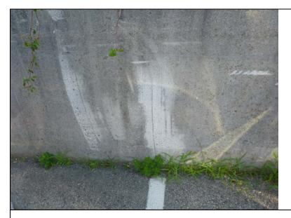
Inspect ID: NAR1\_2019\_a\_0017 Title: USACE\_CENAN\_NAR1\_2019\_a\_0017\_1.jpg Rated Item: 4. Concrete Surfaces Caption: Rating: Minimally Acceptable; Remarks: Gouging of the protected side of monoliths 54-56, may be the result of improper snow removal practices.; Action: The local sponsor should contact the property owner and advise them that the wall cannot be used as a push wall.; Station\_1: 3+50B
