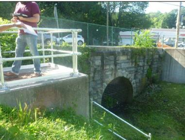
Inspect ID: NAR1\_2019\_a\_0009 Title: USACE\_CENAN\_NAR1\_2019\_a\_0009\_1.jpg Rated Item: 2. Encroachments Caption: Rating: Minimally Acceptable; Remarks: Safety railing installed on the top of Junction Chamber #1 to comply with new OSHA regulations.; Action: Seek authorization for the new railing from USACE.; Station\_1: 4+25B
