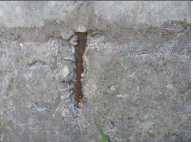
Inspect ID: NAR1\_2019\_a\_0027 Title: USACE\_CENAN\_NAR1\_2019\_a\_0027\_2.jpg Rated Item: 4. Concrete Surfaces Caption: Rating: Minimally Acceptable; Remarks: Exposed rebar near base of monolith 47.; Action: Repair concrete surface in accordance with USACE guidelines.; Station\_1: 2+15B
