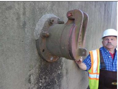
**Inspect ID:** NAR1\_2019\_a\_0052 **Title:** USACE\_CENAN\_NAR1\_2019\_a\_0052\_4.jpg **Rated Item:** 2. Encroachments **Caption:** Rating: Minimally Acceptable; Remarks: Unauthorized flap gate in monolith 18 is connected to 8" IDP noted in observation #50. Flap gate found in open position in 2016.; Action: Maintian flap gate. Investigate easement agreement and dispose of encroachment accordingly.; Station\_1: 3+75U; Photo taken prior to the 2019 inspection.
