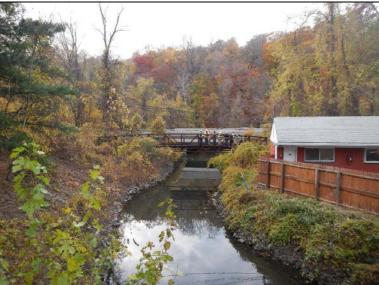
Inspect ID: NAR1\_2019\_a\_0093 Title: USACE\_CENAN\_NAR1\_2019\_a\_0093\_1.jpg Rated Item: 3. Encroachments Caption: Rating: Minimally Acceptable; Remarks: Pedestrian bridge over Saw Mill River replaced the railroad bridge that was to be removed. It is not on the project plans.; Action: Document bridge and verify hydraulics of the river are unaffected.; Station\_1: 0+50D; Photo taken prior to the 2019 inspection.
