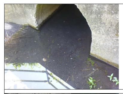
Inspect ID: NAR1\_2019\_a\_0047 Title: USACE\_CENAN\_NAR1\_2019\_a\_0047\_1.jpg Rated Item: 1. Vegetation and Obstructions Caption: Rating: Minimally Acceptable; Remarks: Inlet to Ponding Area #2 (Outlet Structure #1) partially obstructed by sediment. Safety rails have been added to the top of the outlet structure to comply with new OSHA guidelines.; Action: Remove sediment from outlet. Seek authorization for railing from USACE.; Station\_1: 5+15U
