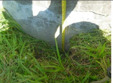
Inspect ID: NAR1\_2019\_a\_0031 Title: USACE\_CENAN\_NAR1\_2019\_a\_0031\_1.jpg Rated Item: 2. Encroachments Caption: Rating: Minimally Acceptable; Remarks: Animal burrow at the base of the protected side of monolith 41. 1 ft deep. 2 ft wide.; Action: Fill the burrow and establish a program to control animal activity near the floodwall.; Station\_1: 8+00 U
