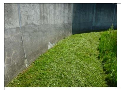
Inspect ID: NAR1\_2019\_a\_0029 Title: USACE\_CENAN\_NAR1\_2019\_a\_0029\_1.jpg Rated Item: 4. Concrete Surfaces Caption: Rating: Minimally Acceptable; Remarks: Concrete spalling on recently repaired areas on the protected side of the floodwall at the base of monoliths 39-42. Exposed rebar on 42. Heavy efflorescence on 41.; Action: Fill cracks and repair spalling in accordance with USACE guidelines.; Station\_1: 0+30B
