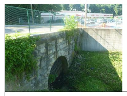
Inspect ID: NAR1\_2019\_a\_0007 Title: USACE\_CENAN\_NAR1\_2019\_a\_0007\_1.jpg Rated Item: 1. Unwanted Vegetation Growth Caption: Rating: Minimally Acceptable; Remarks: Vegetation growth in joints of masonry facade of monolith 59/60. According to NYSDEC, the masonry structure belongs to New York City DEP.; Action: Clean and repoint masonry.; Station 1: 4+45B
