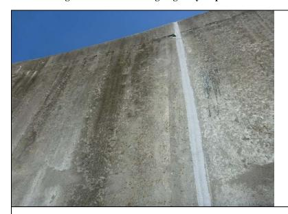
Inspect ID: NAR1\_2019\_a\_0032 Title: USACE\_CENAN\_NAR1\_2019\_a\_0032\_1.jpg Rated Item: 4. Concrete Surfaces Caption: Rating: Minimally Acceptable; Remarks: Apparent construction joint has opened along the top of the protected side of monoliths 39 and 40.; Action: Fill the crack and repair concrete surface in accordance with USACE guidelines.; Station\_1: 7+80U
