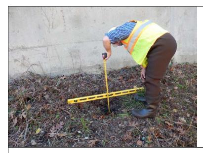
**Inspect ID:** NAR1\_2019\_a\_0020 **Title:** USACE\_CENAN\_NAR1\_2019\_a\_0020\_1.jpg **Rated Item:** 7. Foundation of Concrete Structures **Caption:** Rating: Minimally Acceptable; Remarks: Two large animal burrows on unprotected side of floodwall, 1-2 ft deep. Did not access in 2019.; Action: Eliminate burrowing animals; completely fill in burrows in accordance with USACE guidelines.; Station\_1: 3+30B; Photo taken prior to the 2019 inspection.
