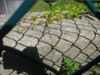
Inspect ID: NAR1\_2019\_a\_0010 Title: USACE\_CENAN\_NAR1\_2019\_a\_0010\_2.jpg Rated Item: 4. Concrete Surfaces Caption: Rating: Minimally Acceptable; Remarks: Hairline crack at the top of monolith 59, associated with missing stone facade.; Action: Monitor to ensure that crack does not widen and repair concrete as necessary.; Station\_1: 4+45B
