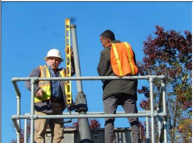
**Inspect ID:** NAR1\_2019\_a\_0043 **Title:** USACE\_CENAN\_NAR1\_2019\_a\_0043\_2.jpg **Rated Item:** 10. Sluice/ Slide Gates **Caption:** Rating: Unacceptable; Remarks: DS#3 valve riser is out of plumb and gate unable to close or operate properly. NYSDEC plans to replace the crank with an electric motor and straighten the gate.; Action: Repair/replace damaged valve riser and restore operation as planned.; Station\_1: 5+15U; Photo taken prior to the 2019 inspection.
