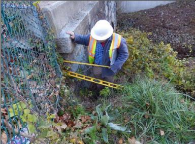
**Inspect ID:** NAR1\_2019\_a\_0003 **Title:** USACE\_CENAN\_NAR1\_2019\_a\_0003\_2.jpg **Rated Item:** 6. Foundation of Concrete Structures **Caption:** Rating: Minimally Acceptable; Remarks: Erosion at headwall on the north side of monolith 60. Vegetation prevented observation in 2019.; Action: Determine source of erosion and repair.; Station\_1: 4+45B; Photo taken prior to 2019 inspection.
