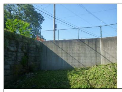
**Inspect ID:** NAR1\_2019\_a\_0004 **Title:** USACE\_CENAN\_NAR1\_2019\_a\_0004\_2.jpg **Rated Item:** 2. Encroachments **Caption:** Rating: Minimally Acceptable; Remarks: Fence on top of floodwall running from monolith 47-60 not in the original plans.; Action: Seek authorization from USACE for the encroachment to remain.; Station\_1: 2+20B; Station\_2: 4+45B
