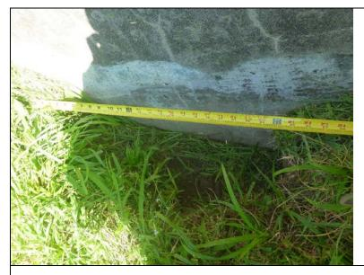
**Inspect ID:** NAR1\_2019\_a\_0031 **Title:** USACE\_CENAN\_NAR1\_2019\_a\_0031\_2.jpg **Rated Item:** 2. Encroachments **Caption:** Rating: Minimally Acceptable; Remarks: Animal burrow at the base of the protected side of monolith 41. 1 ft deep. 2 ft wide.; Action: Fill the burrow and establish a program to control animal activity near the floodwall.; Station\_1: 8+00 U
