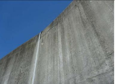
Inspect ID: NAR1\_2019\_a\_0030 Title: USACE\_CENAN\_NAR1\_2019\_a\_0030\_1.jpg Rated Item: 4. Concrete Surfaces Caption: Rating: Minimally Acceptable; Remarks: Spalling near the top of the protected side of monolith 39, near joint with monolith 38..; Action: Fill cracks and repair spalling in accordance with USACE guidelines.; Station\_1: 7+70U; ;;
