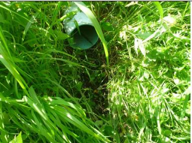
Inspect ID: NAR1\_2019\_a\_0046 Title: USACE\_CENAN\_NAR1\_2019\_a\_0046\_2.jpg Rated Item: 2. Encroachments Caption: Rating: Minimally Acceptable; Remarks: Two 8" PVC pipes that discharge in ponding area #2 are not shown on the project plans. Some erosion has occurred below the southernmost pipe; Action: Local sponsor should investigate and document the encroachments.; Station\_1: 5+15U;
