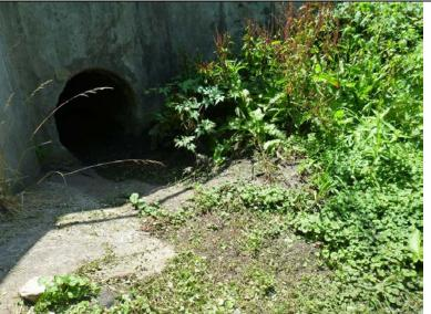
Inspect ID: NAR1\_2019\_a\_0084 Title: USACE\_CENAN\_NAR1\_2019\_a\_0084\_1.jpg Rated Item: 1. Vegetation and Obstructions Caption: Rating: Minimally Acceptable; Remarks: Minor sediment buildup at outlet structure #2.; Action: Remove sediment in accordance with USACE guidelines.; Station\_1: 5+00A;
