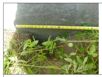
Inspect ID: NAR1\_2019\_a\_0040 Title: USACE\_CENAN\_NAR1\_2019\_a\_0040\_1.jpg Rated Item: 2. Encroachments Caption: Rating: Minimally Acceptable; Remarks: Animal burrow on the protected side at the base of monolith 29. 1 ft deep. 1.5 ft wide.; Action: Fill burrow and establish a program to control animal activity near the flood wall.; Station\_1: 5+80U
