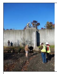
**Inspect ID:** NAR1\_2019\_a\_0043 **Title:** USACE\_CENAN\_NAR1\_2019\_a\_0043\_1.jpg **Rated Item:** 10. Sluice/ Slide Gates **Caption:** Rating: Unacceptable; Remarks: DS#3 valve riser is out of plumb and gate unable to close or operate properly. NYSDEC plans to replace the crank with an electric motor and straighten the gate.; Action: Repair/replace damaged valve riser and restore operation as planned.; Station\_1: 5+15U; Photo taken prior to the 2019 inspection.
