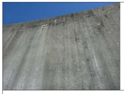
Inspect ID: NAR1\_2019\_a\_0032 Title: USACE\_CENAN\_NAR1\_2019\_a\_0032\_3.jpg Rated Item: 4. Concrete Surfaces Caption: Rating: Minimally Acceptable; Remarks: Apparent construction joint has opened along the top of the protected side of monoliths 39 and 40.; Action: Fill the crack and repair concrete surface in accordance with USACE guidelines.; Station\_1: 7+80U
