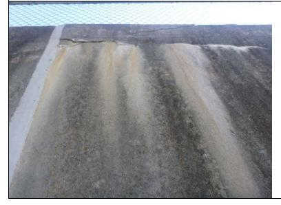
Inspect ID: NAR1\_2019\_a\_0022 Title: USACE\_CENAN\_NAR1\_2019\_a\_0022\_1.jpg Rated Item: 4. Concrete Surfaces Caption: Rating: Minimally Acceptable; Remarks: Crack with efflorescence near the top of the protected side of monolith 51 at the joint with monolith 50.; Action: Repair concrete surface in accordance with USACE Guidelines.; Station\_1: 2+80B
