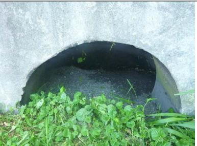
**Inspect ID:** NAR1\_2019\_a\_0001 **Title:** USACE\_CENAN\_NAR1\_2019\_a\_0001\_1.jpg **Rated Item:** 1. Vegetation and Obstructions **Caption:** Rating: Minimally Acceptable; Remarks: Outflow from Junction Chamber # 1 partially blocked with debris and vegetation.; Action: Remove debris and sediment from outlet pipe.; Station\_1: 4+45B
