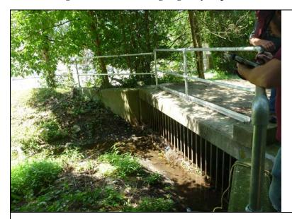
Inspect ID: NAR1\_2019\_a\_0092 Title: USACE\_CENAN\_NAR1\_2019\_a\_0092\_1.jpg Rated Item: 2. Encroachments Caption: Rating: Minimally Acceptable; Remarks: Safety railing installed on top of inlet structure to comply with new OSHA regulations.; Action: Seek authorization from USACE for encroachment.; Station 1: 2+70C
