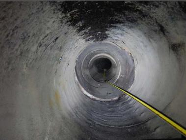
Inspect ID: NAR1\_2019\_a\_0058 Title: USACE\_CENAN\_NAR1\_2019\_a\_0058\_1.jpg Rated Item: 3. Encroachments Caption: Rating: Minimally Acceptable; Remarks: Old drainage inlets at Ardsley Square may not have been properly abandoned. 20" pipe from channel wall remains open. Could not access in 2019.; Action: Confirm that pre-project catch basins were abandoned according to the approved plan.; Station\_1: 1+80U; Photo taken prior to the 2019 inspection.
