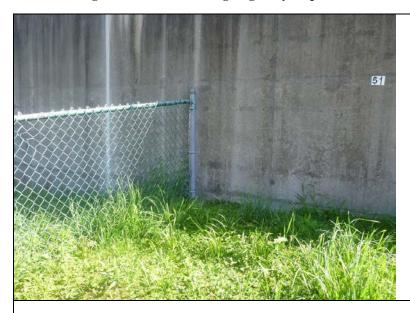
Inspect ID: NAR1\_2019\_a\_0025 Title: USACE\_CENAN\_NAR1\_2019\_a\_0025\_1.jpg Rated Item: 2. Encroachments Caption: Rating: Minimally Acceptable; Remarks: Chain link fence encroaching on protected side of floodwall. Extends 6 ft out from floodwall.; Action: Investigate easement agreement and dispose of encroachment accordingly.; Station\_1: 2+70B
