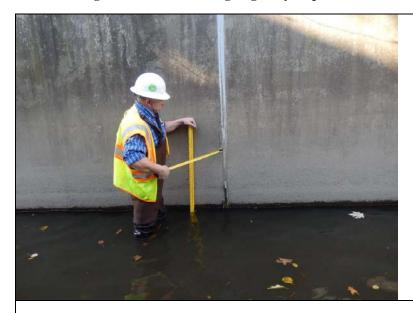
**Inspect ID:** NAR1\_2019\_a\_0056 **Title:** USACE\_CENAN\_NAR1\_2019\_a\_0056\_1.jpg **Rated Item:** 5. Concrete Surfaces **Caption:** Rating: Minimally Acceptable; Remarks: Spalling near joint between monoliths 13 and 14 on the right bank channel wall. Could not access in 2019.; Action: Repair concrete surface in accordance with USACE guidelines.; Station\_1: 2+80U; Photo taken prior to the 2019 inspection.
