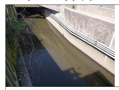
Inspect ID: NAR1\_2019\_a\_0067 Title: USACE\_CENAN\_NAR1\_2019\_a\_0067\_1.jpg Rated Item: 2. Shoaling (sediment deposition) Caption: Rating: Minimally Acceptable; Remarks: Shoaling at DS#1 in flood reduction channel.; Action: Remove sediment from channel to ensure maximum flow capacity.; Station\_1: 0+55U; ;;
