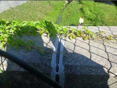
Inspect ID: NAR1\_2019\_a\_0016 Title: USACE\_CENAN\_NAR1\_2019\_a\_0016\_3.jpg Rated Item: 7. Monolith Joints Caption: Rating: Minimally Acceptable; Remarks: The gap sealant has cracked and separated in numerous joints along the entire length of the floodwall.; Action: Explore alternative joint stop material that can withstand the area's unique conditions. Clean joint and apply fresh sealant.; Station\_1: 0+00U; Station\_2: 4+45B
