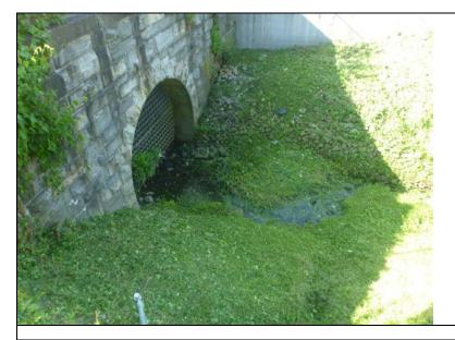
Inspect ID: NAR1\_2019\_a\_0008 Title: USACE\_CENAN\_NAR1\_2019\_a\_0008\_1.jpg Rated Item: 2. Shoaling (sediment deposition) Caption: Rating: Minimally Acceptable; Remarks: Some light sediment at outlet of NYCDEP blow off tunnel.; Action: Remove sediment in accordance with USACE guidelines.; Station\_1: 4+40B
