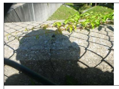
Inspect ID: NAR1\_2019\_a\_0010 Title: USACE\_CENAN\_NAR1\_2019\_a\_0010\_1.jpg Rated Item: 4. Concrete Surfaces Caption: Rating: Minimally Acceptable; Remarks: Hairline crack at the top of monolith 59, associated with missing stone facade.; Action: Monitor to ensure that crack does not widen and repair concrete as necessary.; Station\_1: 4+45B
