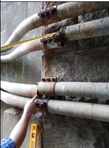
Inspect ID: NAR1\_2019\_a\_0063 Title: USACE\_CENAN\_NAR1\_2019\_a\_0063\_1.jpg Rated Item: 3. Encroachments Caption: Rating: Minimally Acceptable; Remarks: Conduits running along right side of channel are broken under bridge. Could not observe in 2019.; Action: Investigate authorization and have utility owner repair or remove.; Station\_1: 1+35U; Photo taken prior to the 2019 inspection.
