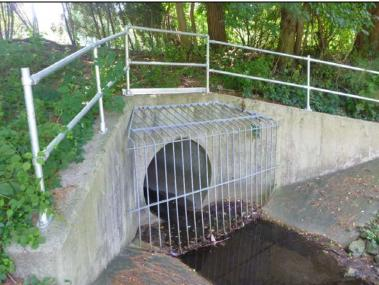
Inspect ID: NAR1\_2019\_a\_0091 Title: USACE\_CENAN\_NAR1\_2019\_a\_0091\_1.jpg Rated Item: 2. Encroachments Caption: Rating: Minimally Acceptable; Remarks: Safety railing installed on top of outlet structure to comply with new OSHA regulations. Minor sediment build up.; Action: Seek authorization from USACE for encroachment. Remove debris and sediment from outlet.; Station\_1: 1+00C
