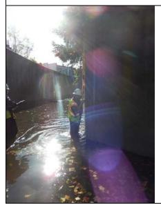
**Inspect ID:** NAR1\_2019\_a\_0077 **Title:** USACE\_CENAN\_NAR1\_2019\_a\_0077\_1.jpg **Rated Item:** 6. Tilting, Sliding or Settlement of Concrete Structures **Caption:** Rating: Minimally Acceptable; Remarks: Right channel wall tilting toward channel 1/4" over 4', between monolith 21 and 22. Could not access in 2019.; Action: Monitor displacement of the concrete monoliths to determine if movement is active.; Station\_1: 4+35U; Photo taken prior to the 2019 inspection.
