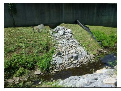
Inspect ID: NAR1\_2019\_a\_0079 Title: USACE\_CENAN\_NAR1\_2019\_a\_0079\_1.jpg Rated Item: 3. Encroachments Caption: Rating: Minimally Acceptable; Remarks: NYCDEC plans to install over the wall piping at monolith 53 for pumps in Ponding Area #2. They have already installed new riprap at the planned outfall to prevent erosion.; Action: Ensure that NYSDEC has authorization from USACE to make these alterations.; Station 1: 3+35B
