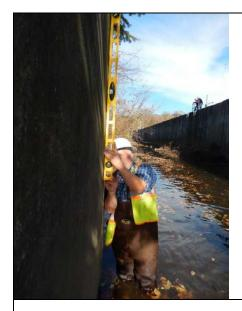
Inspect ID: NAR1\_2019\_a\_0077 Title: USACE\_CENAN\_NAR1\_2019\_a\_0077\_2.jpg Rated Item: 6. Tilting, Sliding or Settlement of Concrete Structures Caption: Rating: Minimally Acceptable; Remarks: Right channel wall tilting toward channel 1/4" over 4', between monolith 21 and 22. Could not access in 2019.; Action: Monitor displacement of the concrete monoliths to determine if movement is active.; Station\_1: 4+35U; Photo taken prior to the 2019 inspection.
