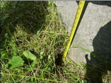
Inspect ID: NAR1\_2019\_a\_0038 Title: USACE\_CENAN\_NAR1\_2019\_a\_0038\_1.jpg Rated Item: 6. Foundation of Concrete Structures Caption: Rating: Minimally Acceptable; Remarks: Animal burrow at base of protected side of monolith 32. 1 ft deep. 1 ft wide.; Action: Fill burrow and establish a program to control animal activity near the floodwall.; Station\_1: 6+30U
