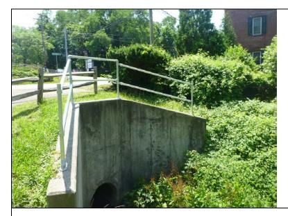
Inspect ID: NAR1\_2019\_a\_0090 Title: USACE\_CENAN\_NAR1\_2019\_a\_0090\_1.jpg Rated Item: 2. Encroachments Caption: Rating: Minimally Acceptable; Remarks: Safety railing installed on top of outlet structure to comply with new OSHA regulations.; Action: Seek authorization from USACE for encroachment.; Station 1: 5+05A
