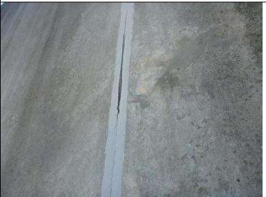
Inspect ID: NAR1\_2019\_a\_0016 Title: USACE\_CENAN\_NAR1\_2019\_a\_0016\_1.jpg Rated Item: 7. Monolith Joints Caption: Rating: Minimally Acceptable; Remarks: The gap sealant has cracked and separated in numerous joints along the entire length of the floodwall.; Action: Explore alternative joint stop material that can withstand the area's unique conditions. Clean joint and apply fresh sealant.; Station\_1: 0+00U; Station\_2: 4+45B
