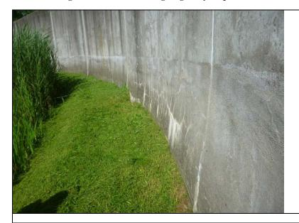
Inspect ID: NAR1\_2019\_a\_0029 Title: USACE\_CENAN\_NAR1\_2019\_a\_0029\_3.jpg Rated Item: 4. Concrete Surfaces Caption: Rating: Minimally Acceptable; Remarks: Concrete spalling on recently repaired areas on the protected side of the floodwall at the base of monoliths 39-42. Exposed rebar on 42. Heavy efflorescence on 41.; Action: Fill cracks and repair spalling in accordance with USACE guidelines.; Station\_1: 0+30B
