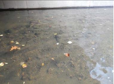
Inspect ID: NAR1\_2019\_a\_0064 Title: USACE\_CENAN\_NAR1\_2019\_a\_0064\_1.jpg Rated Item: 2. Shoaling (sediment deposition) Caption: Rating: Minimally Acceptable; Remarks: Shoaling at bottom of channel at south side of old bridge. Could not observe through high water in 2019.; Action: Remove sediment from channel to ensure maximum flow capacity.; Station\_1: 1+35U; Photo taken prior to the 2019 inspection.
