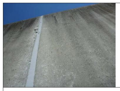
Inspect ID: NAR1\_2019\_a\_0039 Title: USACE\_CENAN\_NAR1\_2019\_a\_0039\_1.jpg Rated Item: 4. Concrete Surfaces Caption: Rating: Minimally Acceptable; Remarks: Small spall on the protected side of monolith 28 at the joint with monolith 29.; Action: Repair concrete surface in accordance with USACE guidelines.; Station\_1: 5+65U
