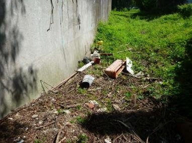
**Inspect ID:** NAR1\_2019\_a\_0055 **Title:** USACE\_CENAN\_NAR1\_2019\_a\_0055\_1.jpg **Rated Item:** 1. Vegetation and Obstructions **Caption:** Rating: Minimally Acceptable; Remarks: Overland drainage on the protected side of the floodwall at monolith 12/13 blocked with debris and sediment.; Action: Restore overland drainage.; Station\_1: 2+50U
