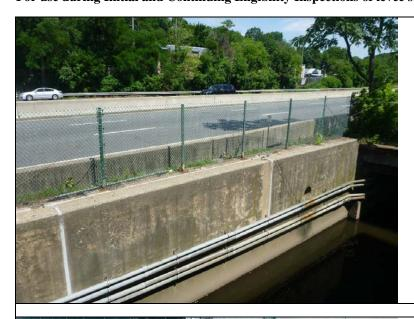
Inspect ID: NAR1\_2019\_a\_0068 Title: USACE\_CENAN\_NAR1\_2019\_a\_0068\_1.jpg Rated Item: 3. Encroachments Caption: Rating: Minimally Acceptable; Remarks: A chain metal fence on the wall of the right bank is not on as-built plans.; Action: Investigate easement agreement and dispose of fence encroachment accordingly.; Station\_1: 0+55U
