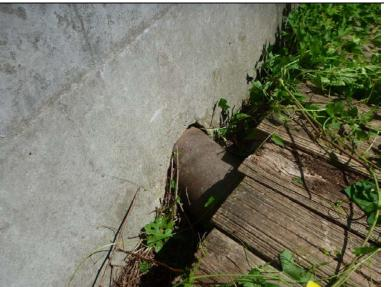
Inspect ID: NAR1\_2019\_a\_0050 Title: USACE\_CENAN\_NAR1\_2019\_a\_0050\_1.jpg Rated Item: 2. Encroachments Caption: Rating: Minimally Acceptable; Remarks: Unauthorized ductile iron pipe through floodwall monolith 18 not on approved plans. Has flap gate but it was found open in 2016.; Action: Maintain flap gate. Investigate easement agreement and dispose of encroachment accordingly.; Station\_1: 3+75U
