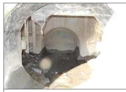
Inspect ID: NAR1\_2019\_a\_0034 Title: USACE\_CENAN\_NAR1\_2019\_a\_0034\_2.jpg Rated Item: 10. Sluice/ Slide Gates Caption: Rating: Minimally Acceptable; Remarks: DS # 4 sluice gate operated during 2016 inspection. Cannot fully close due to sediment at bottom of structure. NYSDEC plans to replace the crank with an electric motor.; Action: Remove sediment and debris.; Station\_1: 6+85U; ;; Photo taken prior to 2019 inspection.
