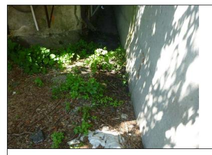
Inspect ID: NAR1\_2019\_a\_0055 Title: USACE\_CENAN\_NAR1\_2019\_a\_0055\_2.jpg Rated Item: 1. Vegetation and Obstructions Caption: Rating: Minimally Acceptable; Remarks: Overland drainage on the protected side of the floodwall at monolith 12/13 blocked with debris and sediment.; Action: Restore overland drainage.; Station\_1: 2+50U
