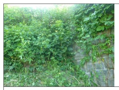
**Inspect ID:** NAR1\_2019\_a\_0003 **Title:** USACE\_CENAN\_NAR1\_2019\_a\_0003\_1.jpg **Rated Item:** 6. Foundation of Concrete Structures **Caption:** Rating: Minimally Acceptable; Remarks: Erosion at headwall on the north side of monolith 60. Vegetation prevented observation in 2019.; Action: Determine source of erosion and repair.; Station\_1: 4+45B
