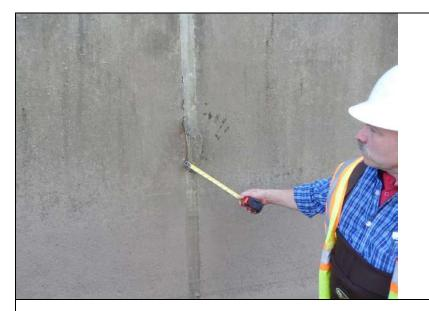
Inspect ID: NAR1\_2019\_a\_0051 Title: USACE\_CENAN\_NAR1\_2019\_a\_0051\_1.jpg Rated Item: 4. Concrete Surfaces Caption: Rating: Minimally Acceptable; Remarks: Spalling on the unprotected side of flood wall near joint between monoliths 21 and 20. Could not access in 2019.; Action: Repair concrete surface in accordance with USACE Guidelines.; Station\_1: 3+85U; Photo taken prior to the 2019 inspection.
