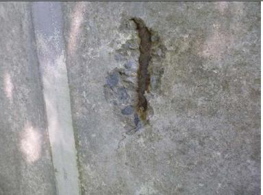
Inspect ID: NAR1\_2019\_a\_0049 Title: USACE\_CENAN\_NAR1\_2019\_a\_0049\_1.jpg Rated Item: 4. Concrete Surfaces Caption: Rating: Minimally Acceptable; Remarks: Minor spall with exposed rebar on the protected side of monolith 24 near the joint with monolith 23.; Action: NA; Station 1: 4+70U
