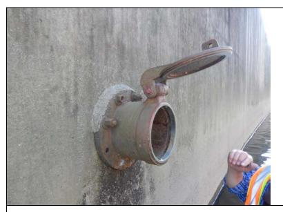
Inspect ID: NAR1\_2019\_a\_0052 Title: USACE\_CENAN\_NAR1\_2019\_a\_0052\_3.jpg Rated Item: 2. Encroachments Caption: Rating: Minimally Acceptable; Remarks: Unauthorized flap gate in monolith 18 is connected to 8" IDP noted in observation #50. Flap gate found in open position in 2016.; Action: Maintian flap gate. Investigate easement agreement and dispose of encroachment accordingly.; Station\_1: 3+75U; Photo taken prior to the 2019 inspection.
