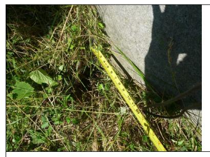
Inspect ID: NAR1\_2019\_a\_0038 Title: USACE\_CENAN\_NAR1\_2019\_a\_0038\_2.jpg Rated Item: 6. Foundation of Concrete Structures Caption: Rating: Minimally Acceptable; Remarks: Animal burrow at base of protected side of monolith 32. 1 ft deep. 1 ft wide.; Action: Fill burrow and establish a program to control animal activity near the floodwall.; Station\_1: 6+30U
