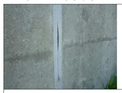
Inspect ID: NAR1\_2019\_a\_0016 Title: USACE\_CENAN\_NAR1\_2019\_a\_0016\_2.jpg Rated Item: 7. Monolith Joints Caption: Rating: Minimally Acceptable; Remarks: The gap sealant has cracked and separated in numerous joints along the entire length of the floodwall.; Action: Explore alternative joint stop material that can withstand the area's unique conditions. Clean joint and apply fresh sealant.; Station\_1: 0+00U; Station\_2: 4+45B
