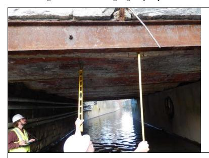
Inspect ID: NAR1\_2019\_a\_0062 Title: USACE\_CENAN\_NAR1\_2019\_a\_0062\_4.jpg Rated Item: 3. Encroachments Caption: Rating: Minimally Acceptable; Remarks: Bricks of the vaulted ceiling, beneath the old bridge, are about to fall due to corroded and broken tie rods. Falling debris could obstruct the channel. Could not observe in 2019.; Action: Shoring is needed to prevent failure of the vaulted ceiling and original bridge structure.; Station\_1: 1+35U; Photo taken prior to the 2019 inspection.
