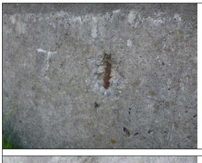
Inspect ID: NAR1\_2019\_a\_0027 Title: USACE\_CENAN\_NAR1\_2019\_a\_0027\_1.jpg Rated Item: 4. Concrete Surfaces Caption: Rating: Minimally Acceptable; Remarks: Exposed rebar near base of monolith 47.; Action: Repair concrete surface in accordance with USACE guidelines.; Station\_1: 2+15B
