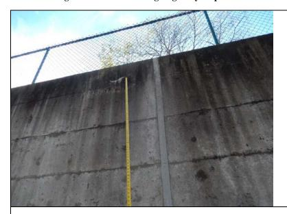
Inspect ID: NAR1\_2019\_a\_0023 Title: USACE\_CENAN\_NAR1\_2019\_a\_0023\_1.jpg Rated Item: 4. Concrete Surfaces Caption: Rating: Minimally Acceptable; Remarks: Spall with efflorescence at top of monolith 51 on the unprotected side. Could not access in 2019.; Action: Repair concrete surface in accordance with USACE Guidelines.; Station\_1: 2+80B; Photo taken prior to the 2019 inspection.
