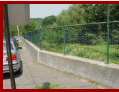
FloodWallalongBlow-offchannel
