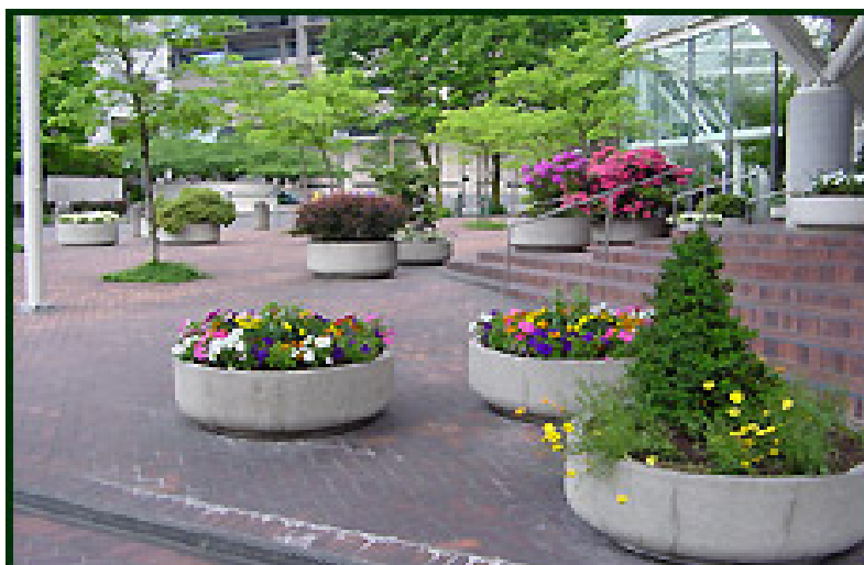
Figure 5.53 Contained stormwater planters made of concrete
