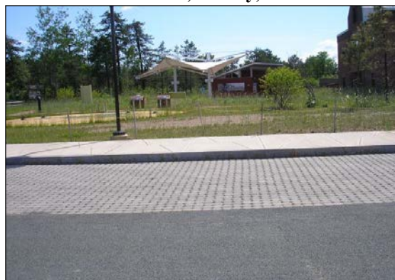
Figure 5.58 Asphalt, Permeable Pavers, Porous Concrete, Albany, NY
