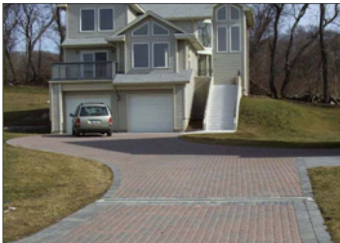
Figure 5.20 Permeable pavers as an alternative driveway surface
